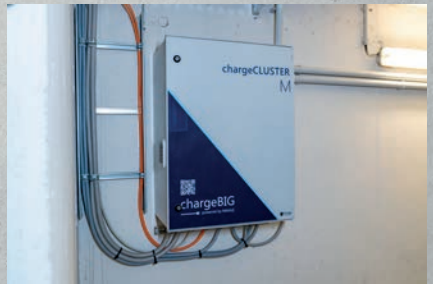
chargeCLUSTER Preconfigured sub-distribution
